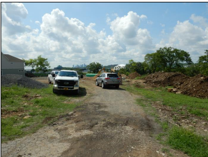
3. Site view, temp drive
