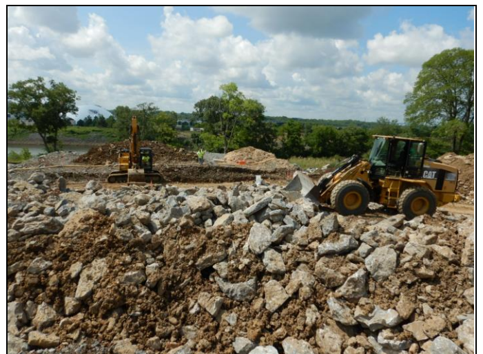
6. Rock removal and fill
