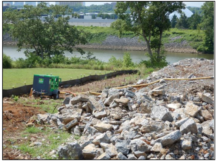
8. Silt fence, rock fill
